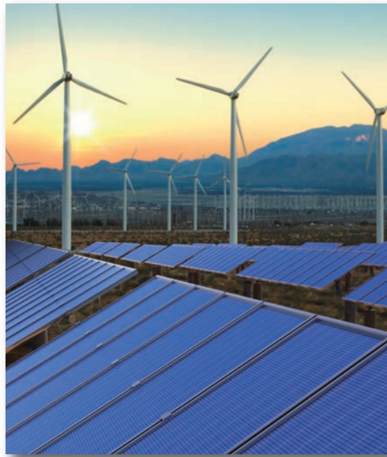
SCADA wind and solar site monitoring
